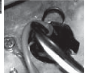
FIG. 5-3 Power cord strain relief
